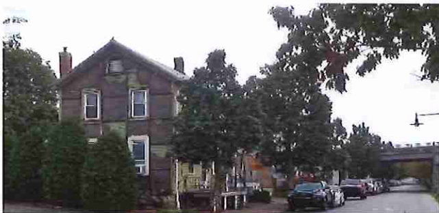
Code enforcement is the proper tool to address a stalled home improvement project and neglected property maintenance.
