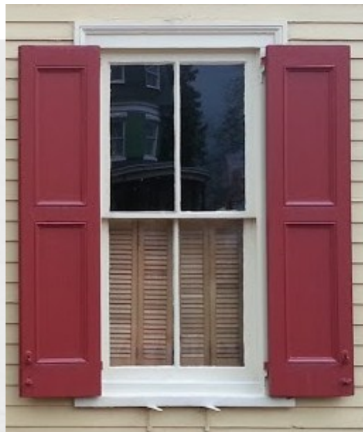
Left—2 over 2, wood, double-hung window with appropriately sized and mounted shutters. Right—6 over 6, wood, double-hung window with wood storm window.
